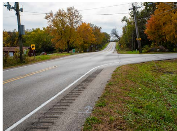
Cary Algonquin Road and Klasen Road intersection looking south.
